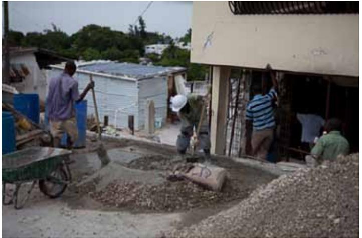
Poorly graded sand and aggregate will result in poor quality concrete. Here it is being used to pour thin columns to support the failing damaged concrete structure above.
