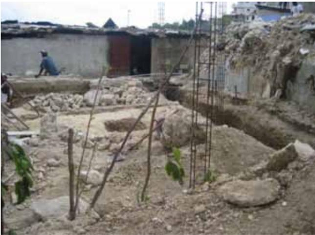
*New construction being set up for a home with typical widely spaced and inadequate vertical reinforcement.*
