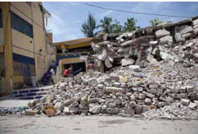
*Large buildings such as this pancaked structure which was once about 4 stories tall are difficult and expensive to build to meet earthquake standards. It is imperative if such structures are to be built, that they must be required to meet international codes and have strict quality control and inspection standards during construction. Imagine the lives lost in just this one building.*
